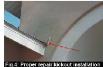
Fig 4: Proper repair kickout installation
