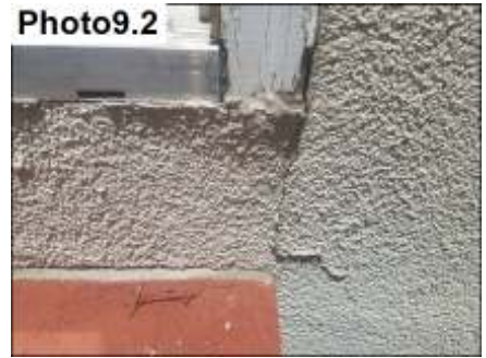
Crack notice below door. Needs repair.
