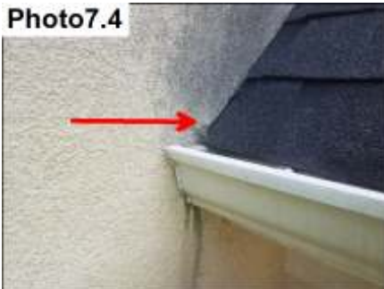
Kickout should be installed here.
