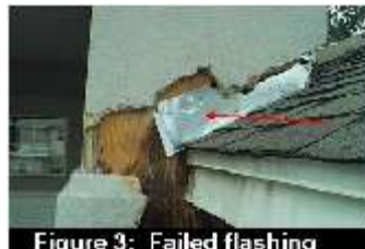
Figure 3: Failed flashing
